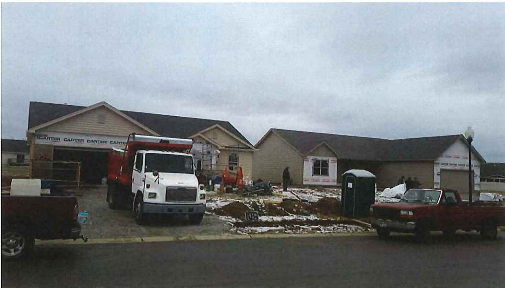
New Single Family Homes under construction in the Timber Glen Subdivision
