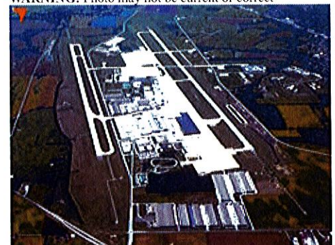
Photo taken 11-Sep-2012 looking west.
