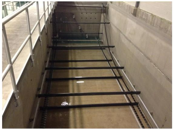
New chains and rakes for sedimentation basin 1-A installed by Water Dept. employees.
